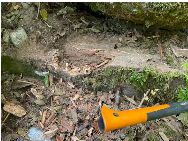
Timber sill condition at right bank
