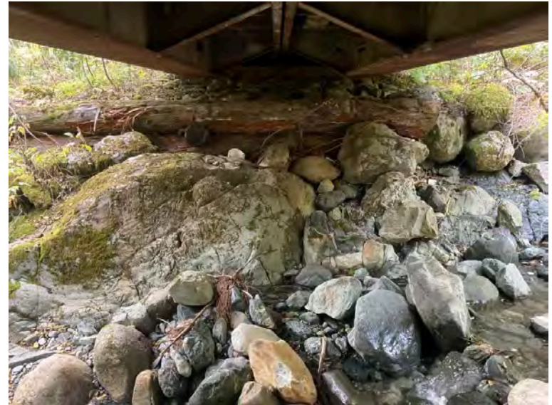
Right Bank Abutment when facing downstream
