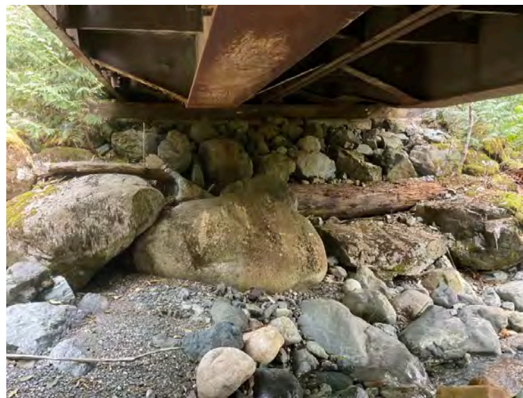
Left Bank Abutment when facing downstream
