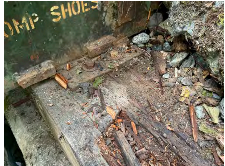
Bearing plate and girder connection
