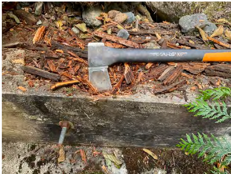
Timber sill condition at left bank
